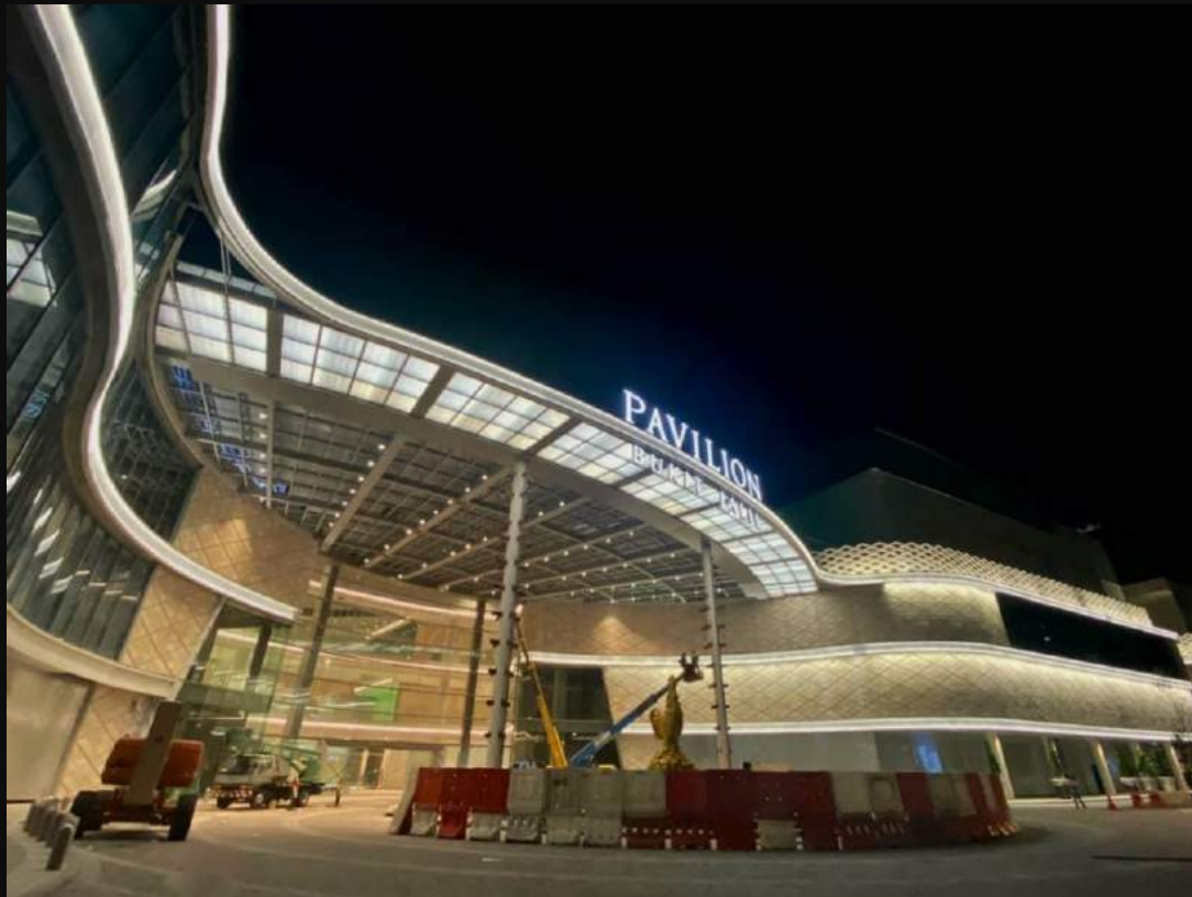
MAIN ENTRANCE CANOPY & UHPC WALL CLADDING
